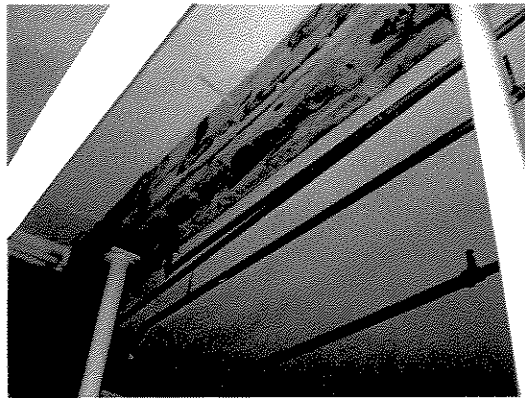
089 Former Fire Station Beams
